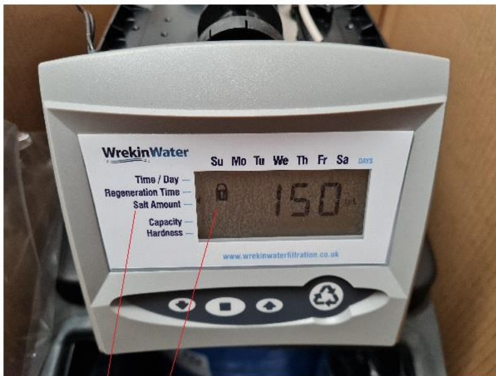
Salt amount Setting - factory set for model and usually locked to prevent accidental changing
